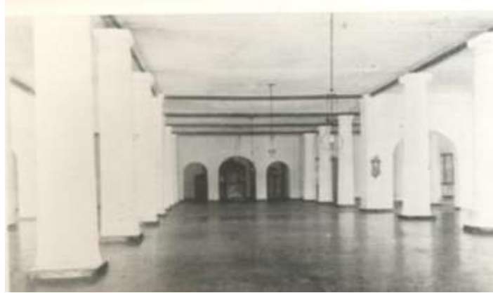
Interior pilar-pilar Masjid Manonjaya (Sumber: Balai Poestaka, 1926)
